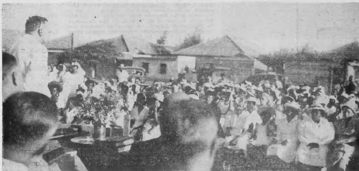
A civic-minded man, Mr. Smith has always been ready to assist any worthy community effort. At left he lays a stone during the cornerstone ceremonies at the new Methodist Church August 1. Above, he addresses the congregation, stating his strong belief in religion's important function of building and sustaining the moral character of a community.
